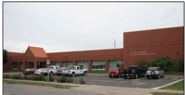
Central Maintenance Facility – 910 Forest Street
