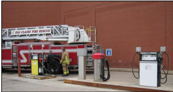
Fuel Pumps at CMF
