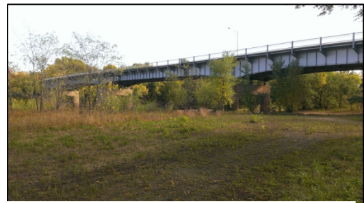
Water Street Bridge
