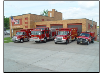
Fire Station No 10, 559 North Hastings Way
