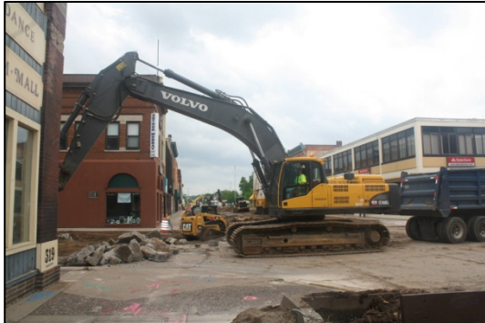
Street reconstruction on Barstow Street
