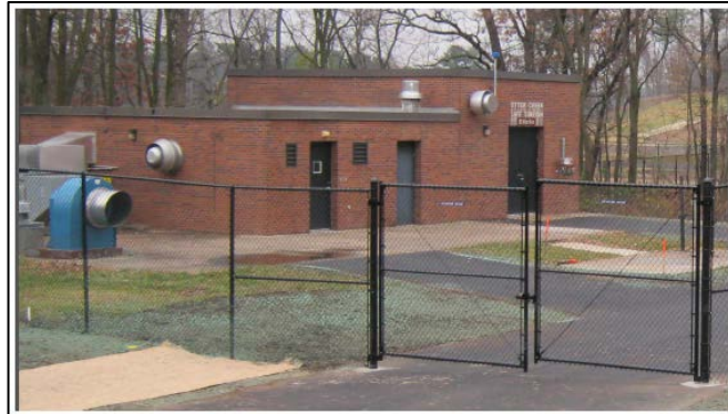
Otter Creek Lift Station
