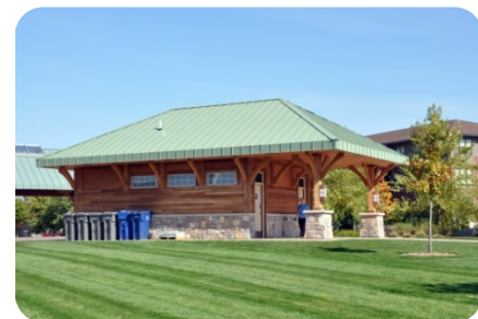
Phoenix Park Restrooms
