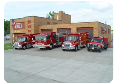
Fire Station No 10, 559 North Hastings Way
