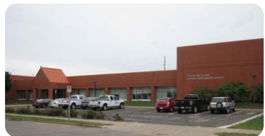
Central Maintenance Facility – 910 Forest Street
