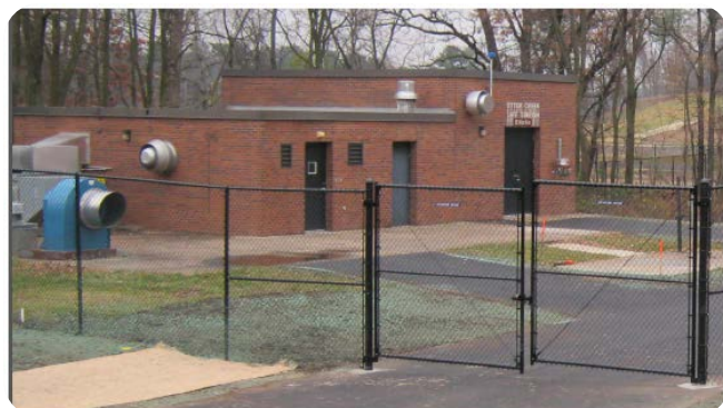
Otter Creek Lift Station
