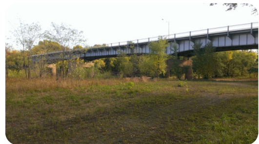
Water Street Bridge
