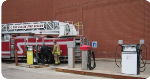
Fuel Pumps at CMF
