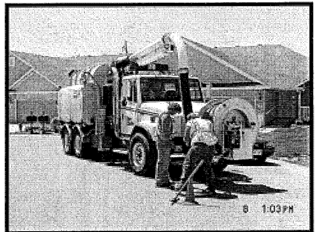
Sanitary Sewer Pipe Cleaning
