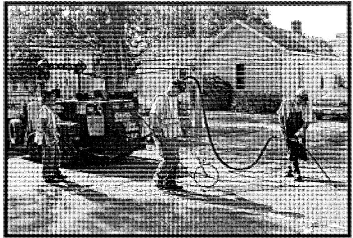
Crack Routing for Crack Sealing Program
