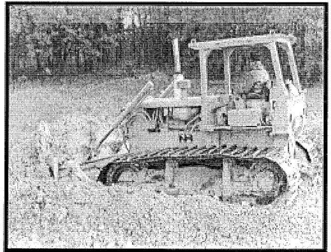
Clay cap at former landfill
