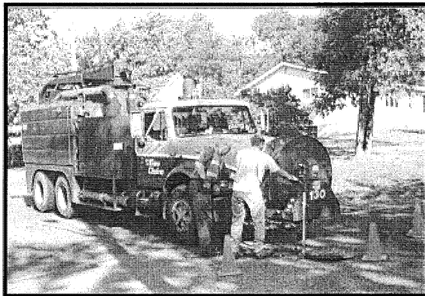
Storm Sewer Pipe Cleaning
