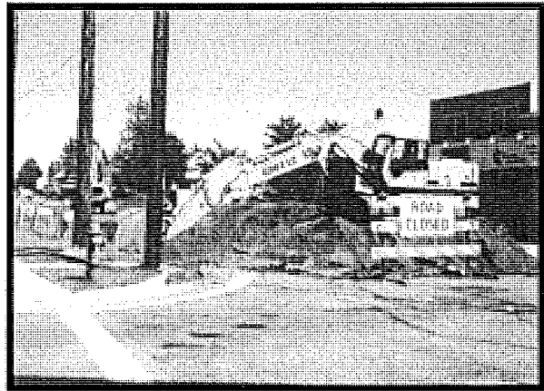
Street & Utility Reconstruction
