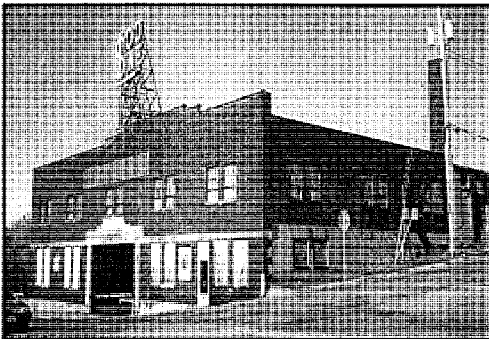
Soo Line site before development project
