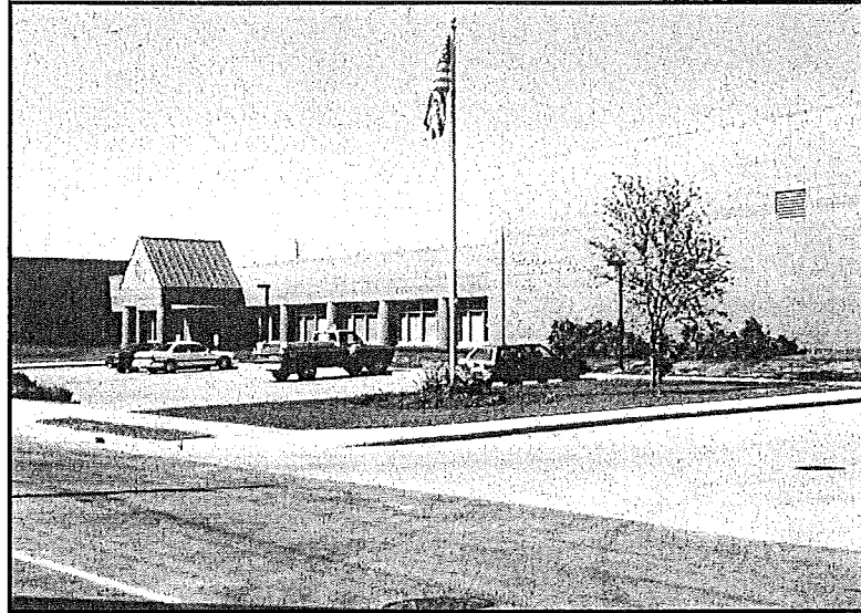
Central Maintenance Facility 910 Forest Street
