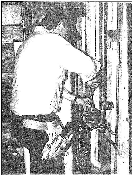
Above: Installing a meter
