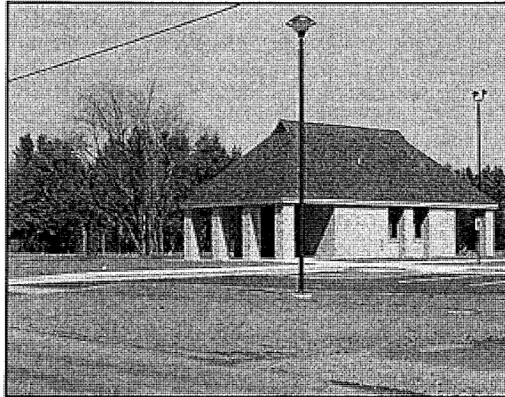
Sundet Road Neighborhood Park Warming House
