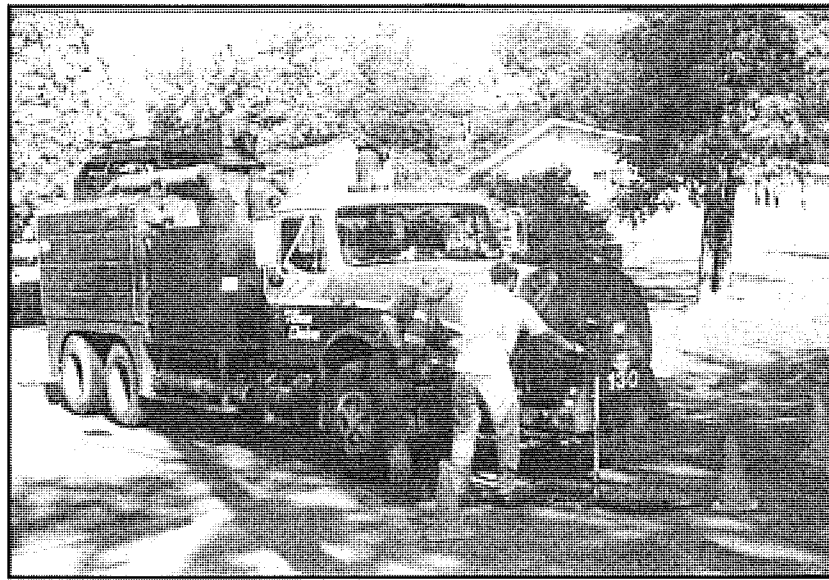
Storm Sewer Pipe Cleaning
