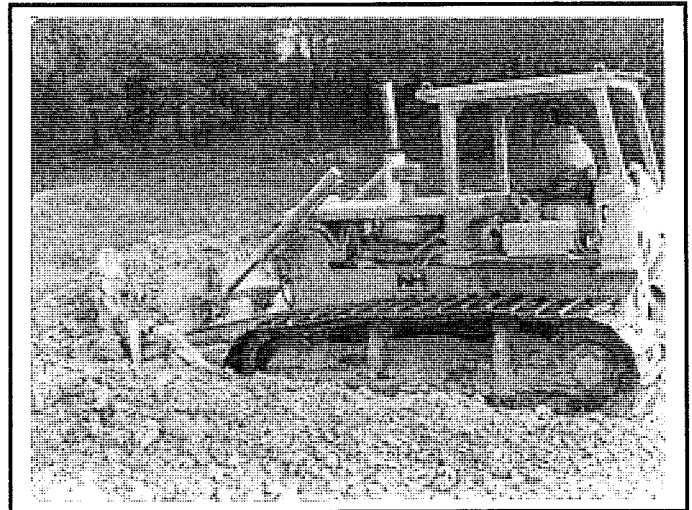
Clay cap at former landfill
