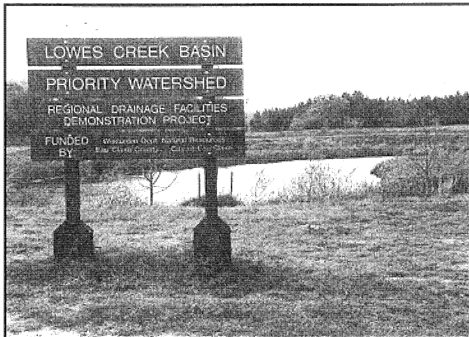
Lowes Creek Detention Basin
