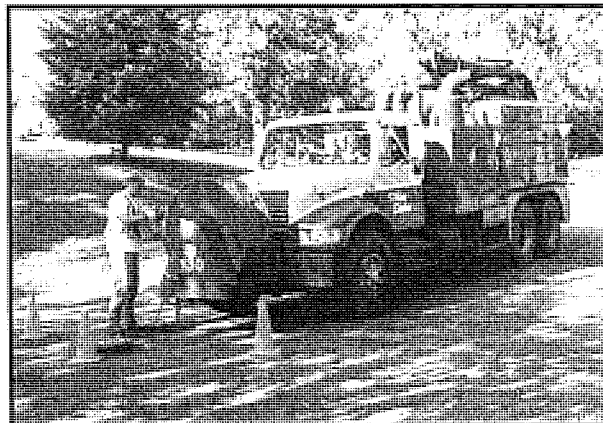
Sanitary Sewer Pipe Cleaning
