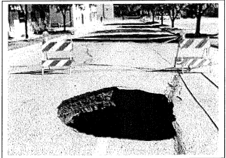
Flood related sinkhole
