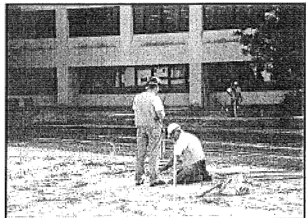
Survey Crew with Geodimeter
