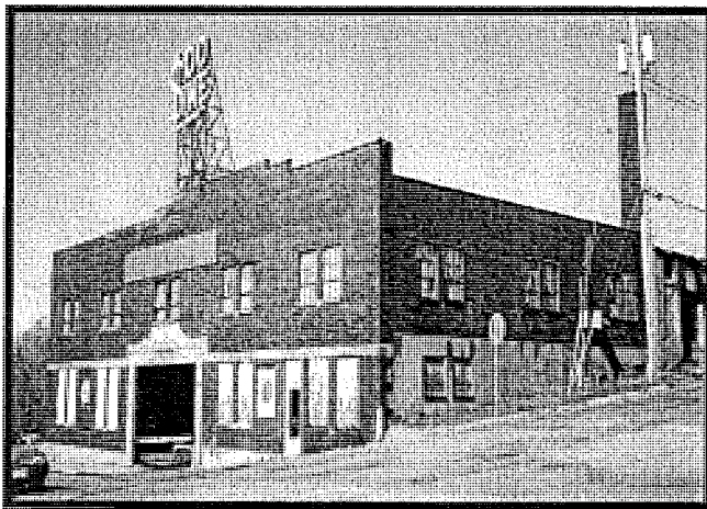
Soo Line site before development project
