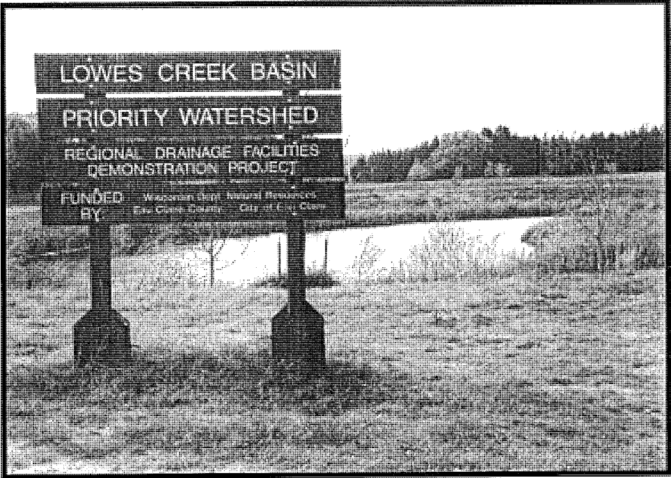
Lowes Creek Detention Basin
