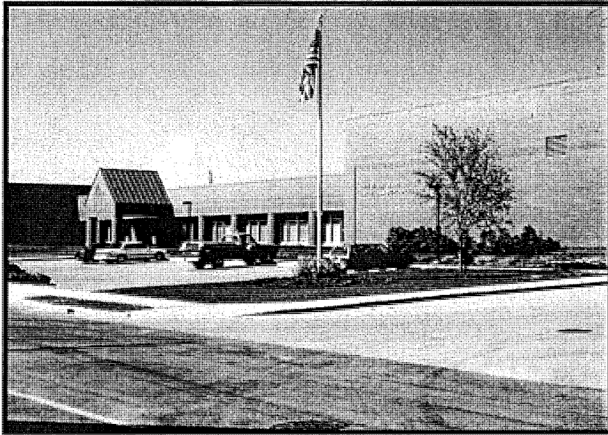
Central Maintenance Facility 910 Forest Street
