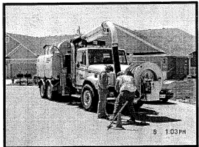
Sanitary Sewer Pipe Cleaning
