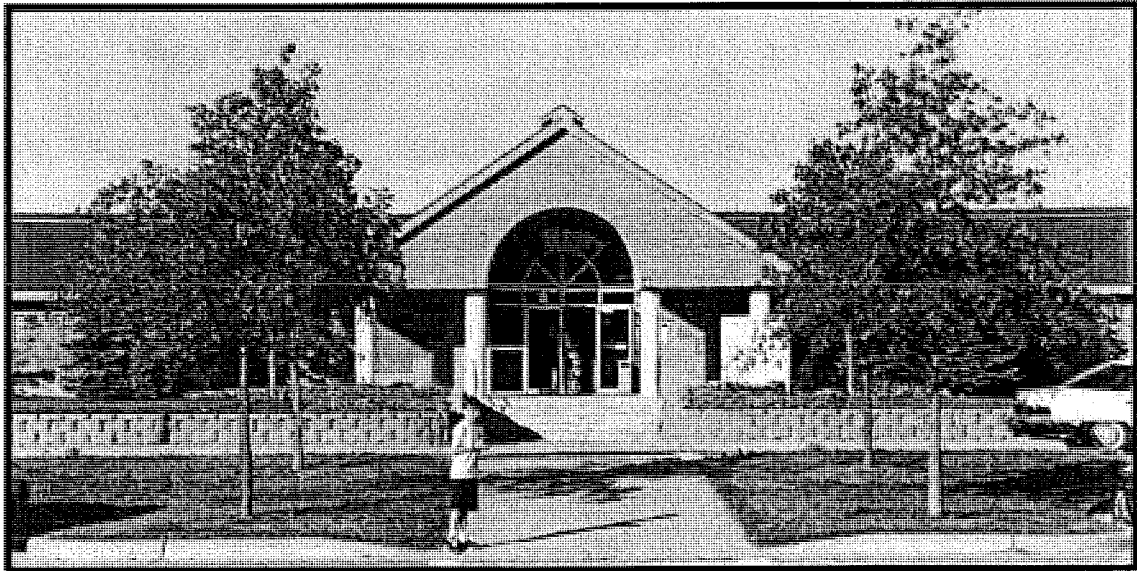
Entrance to Fairfax Pool
