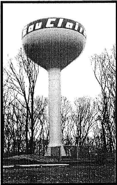
Oakwood Hills Water Tower
