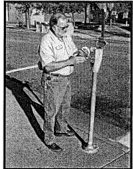
Parking Meter Repairs
