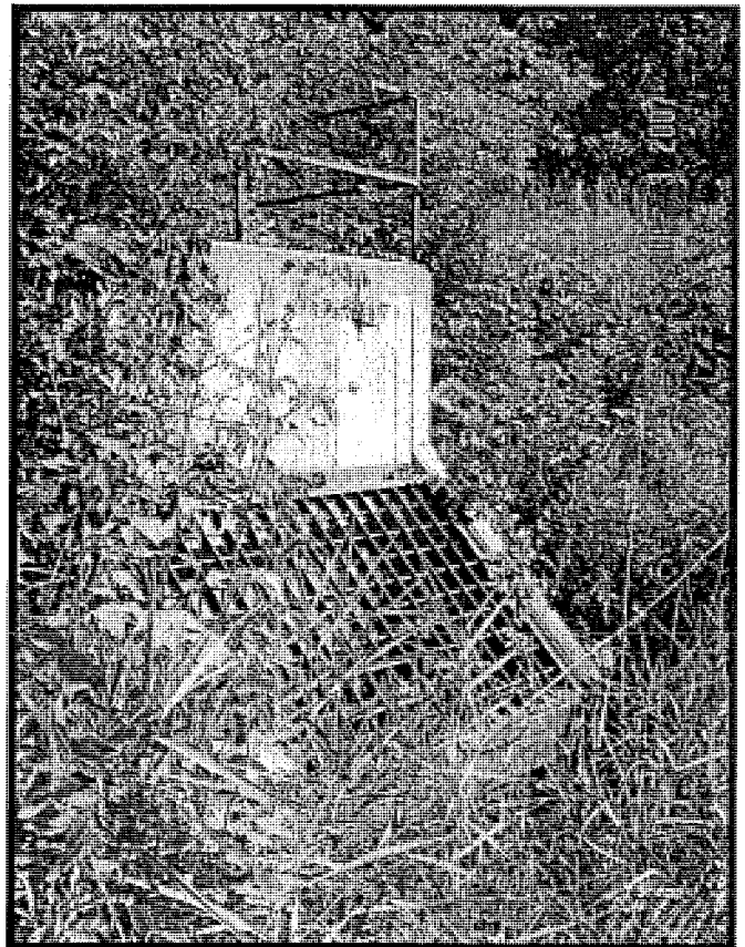
Lowes Creek & Eau Claire County Fairgrounds Outfall Structure
