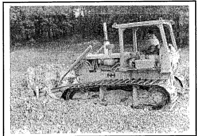
Clay cap at former landfill
