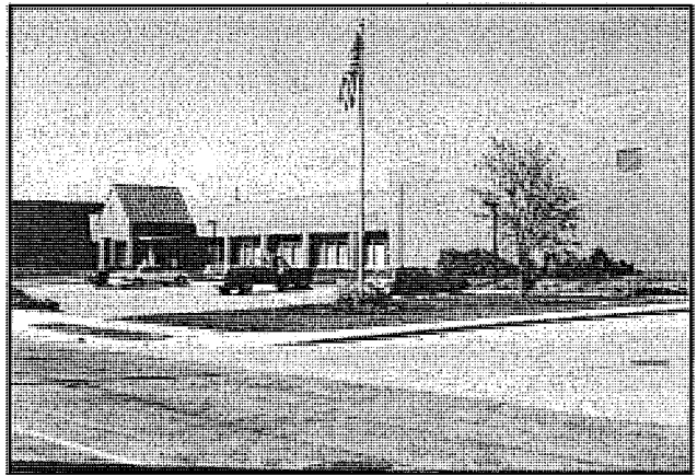
Central Maintenance Facility
