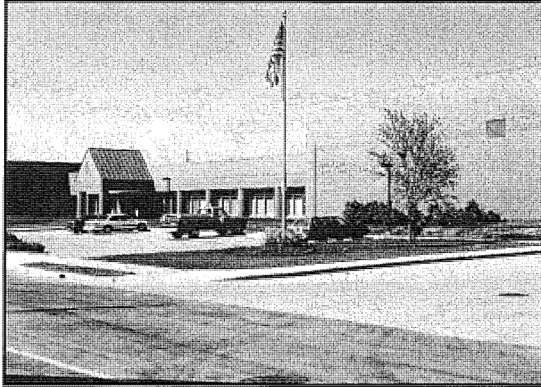
Central Maintenance Facility 910 Forest Street
