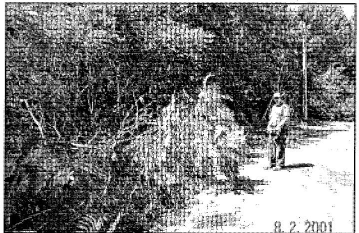
Brush removal along trail
