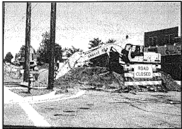
Street & Utility Reconstruction
