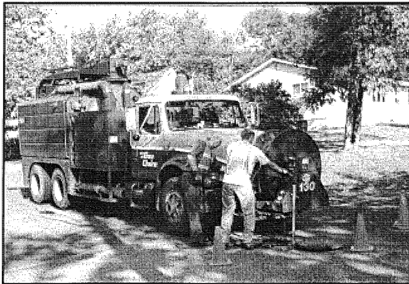
Storm Sewer Pipe Cleaning
