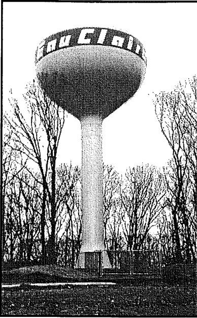
Oakwood Hills Water Tower
