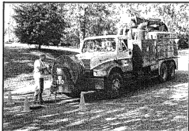
Sanitary Sewer Pipe Cleaning
