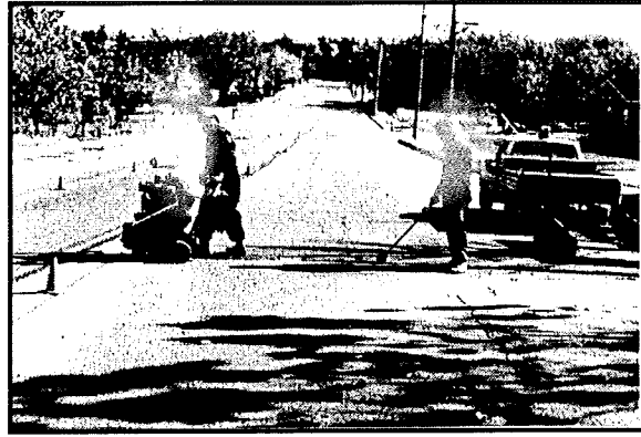
Crack Sealing
