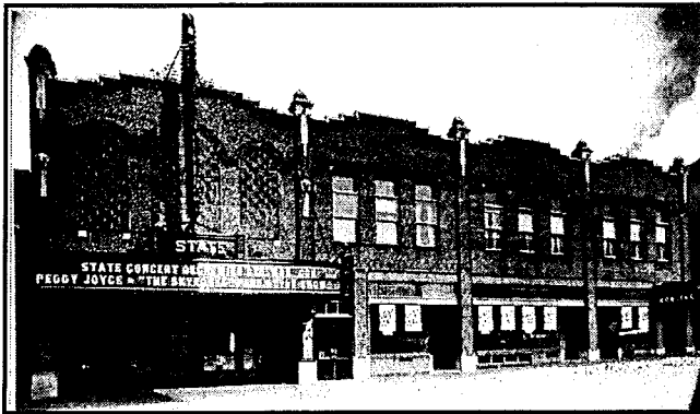
State Theatre Building 1926
