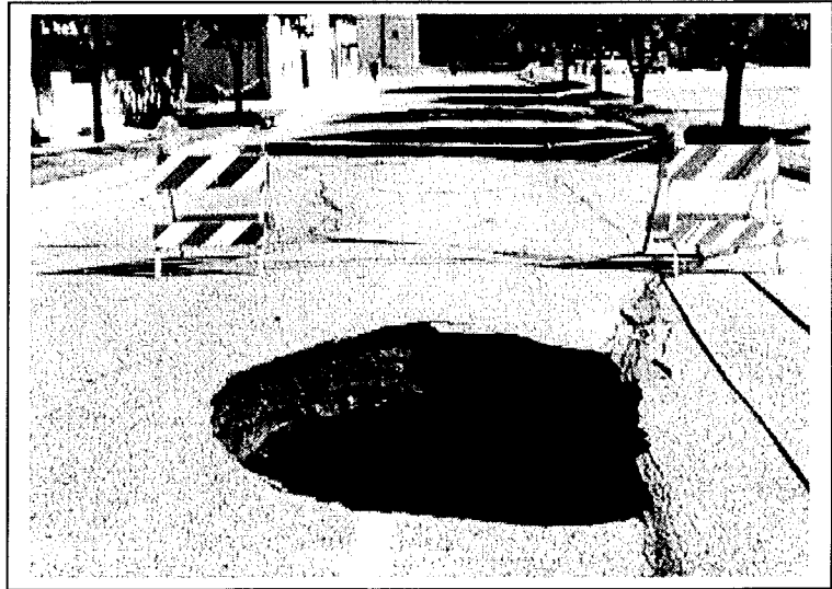
Flood related sinkhole
