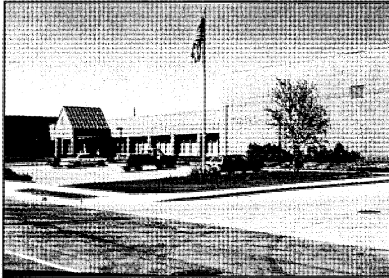
Central Maintenance Facility 910 Forest Street
