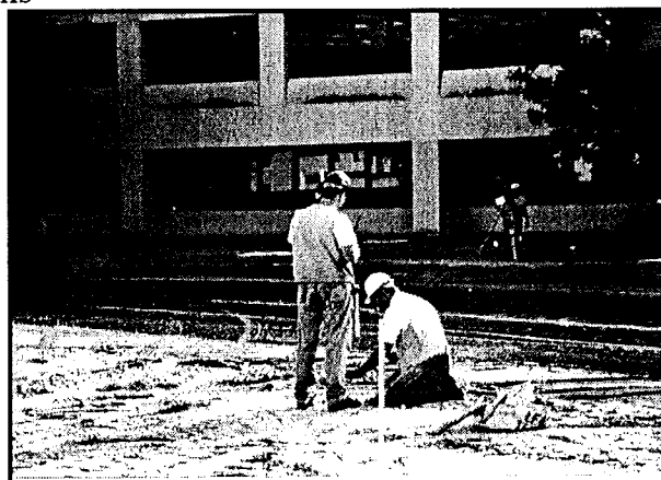
Survey Crew with Geodimeter
