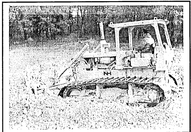
Clay cap at former landfill
