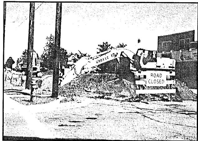
Street & Utility Reconstruction
