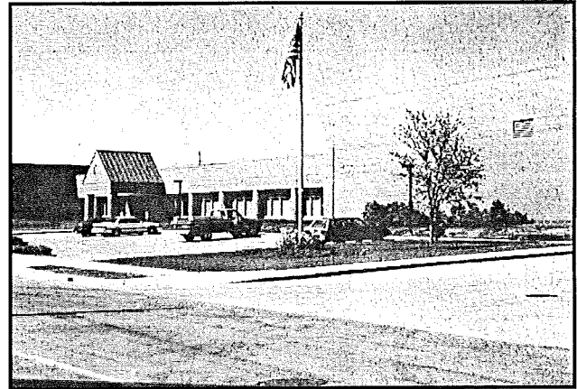
Central Maintenance Facility
