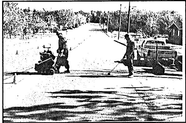
Crack Routing for Crack Sealing Program
