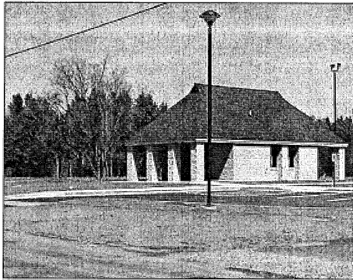
Sundet Road Neighborhood Park Warming House
