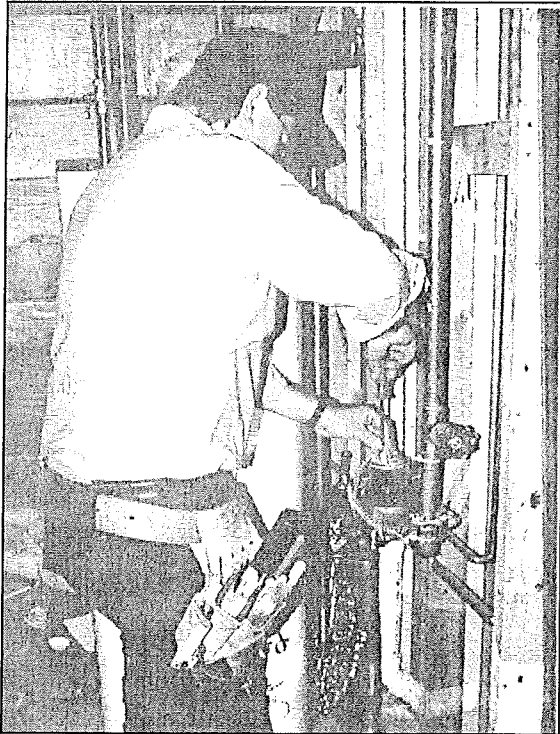
Above: Installing a meter
