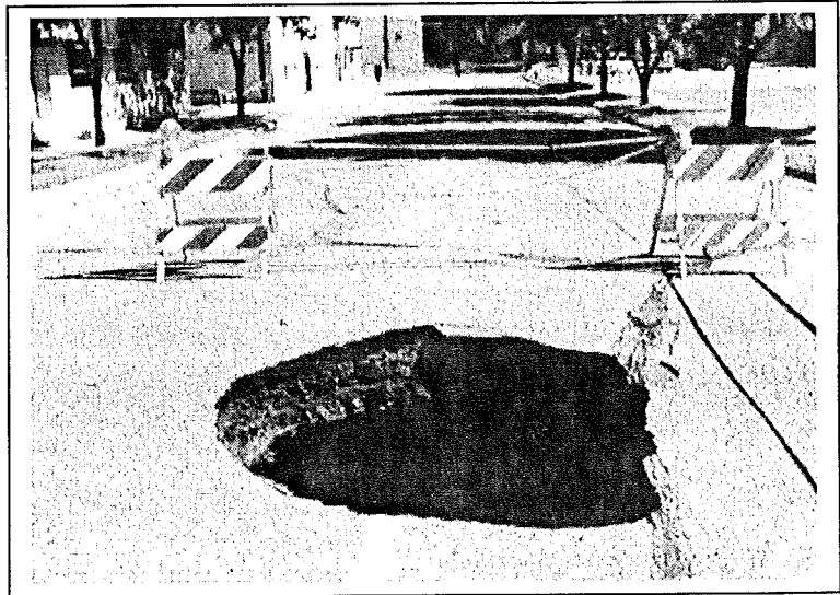
Flood related sinkhole
