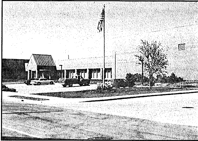
Central Maintenance Facility 910 Forest Street
