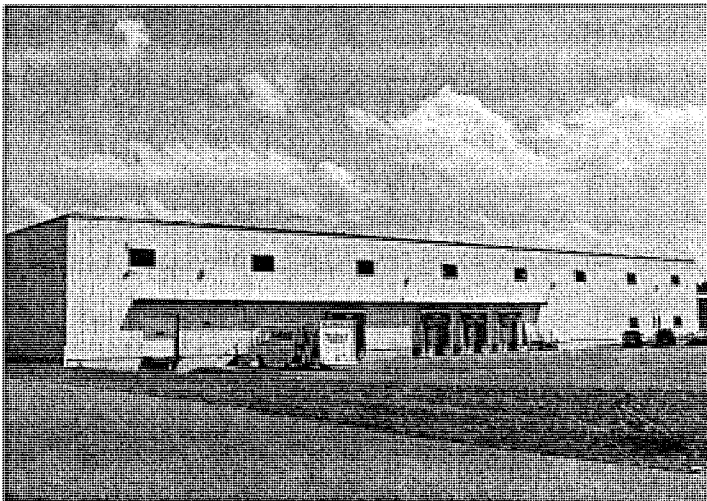
Huebsch Linen expanded their facility by 15,000 square feet in the Chippewa Valley Industrial Park.
