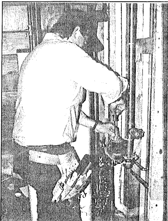
Above: Installing a meter
