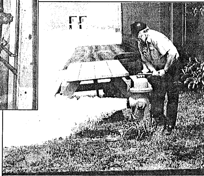
Left: Hydrants are flushed to assure clean water lines.
