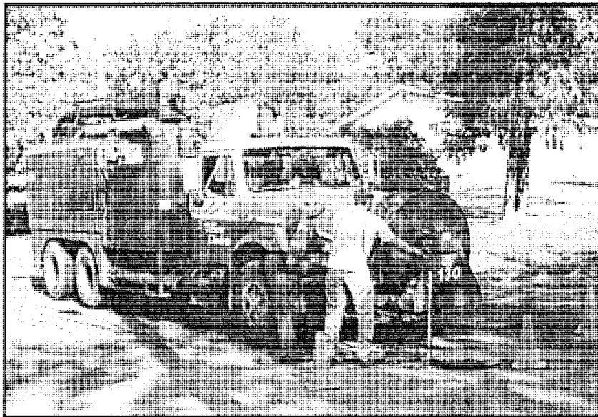
Storm Sewer Pipe Cleaning
