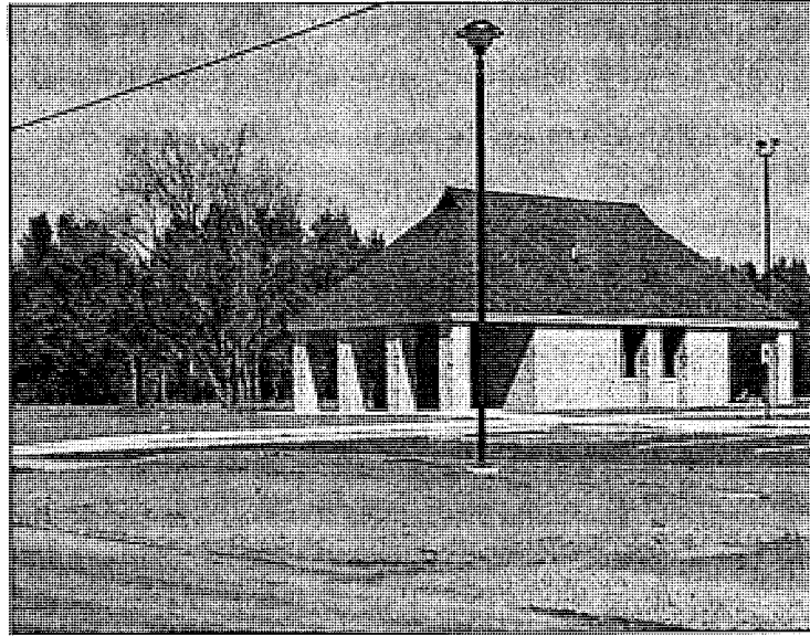
Sundet Road Neighborhood Park Warming House
