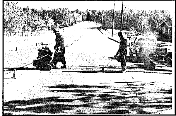
Crack Routing for Crack Sealing Program
