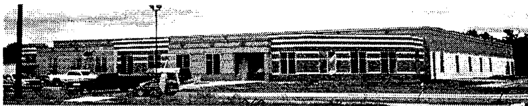
ENCOR Technologies' new facility
