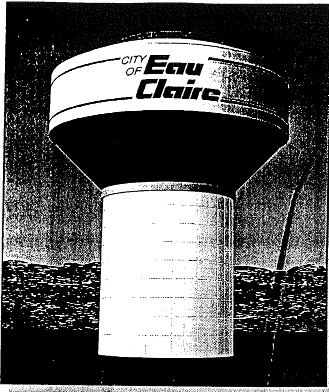
New 2 million gallon water tower on Folsom Street.
