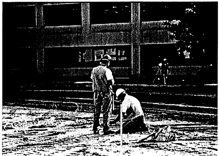
Survey Crew with Geodimeter
