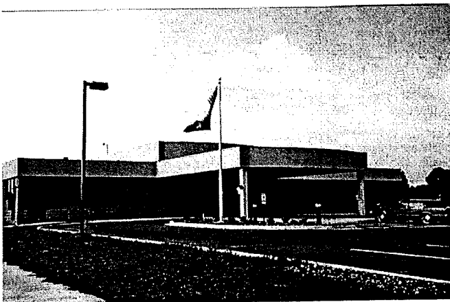
New L.E. Phillips Senior Center – total CDBG contribution over $1 million for land acquisition, clearance and new construction.
