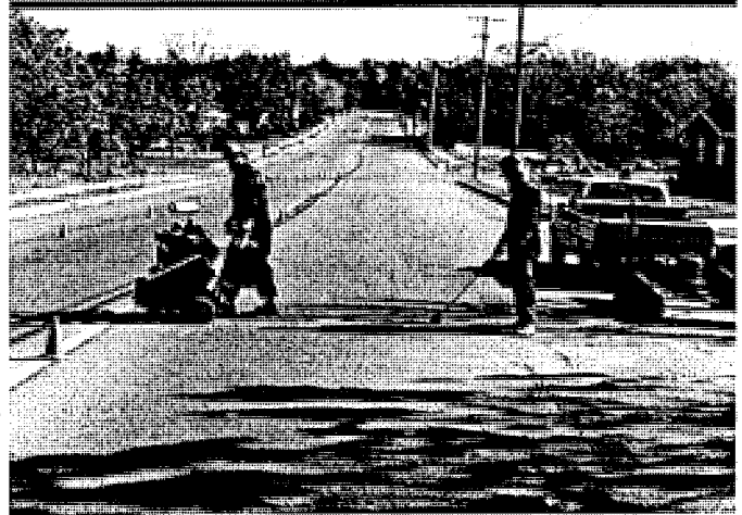
Crack Sealing
