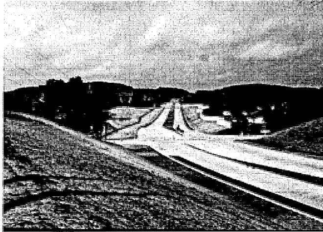
North Crossing Construction
