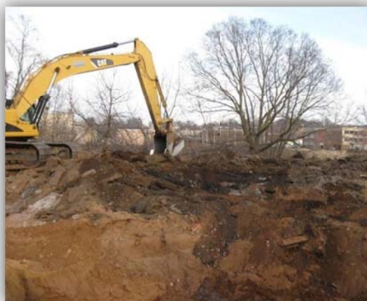
Owen Park Remediation. Xcel Energy Photo
