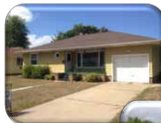
Homeownership Project at 228 E Tyler Ave.
