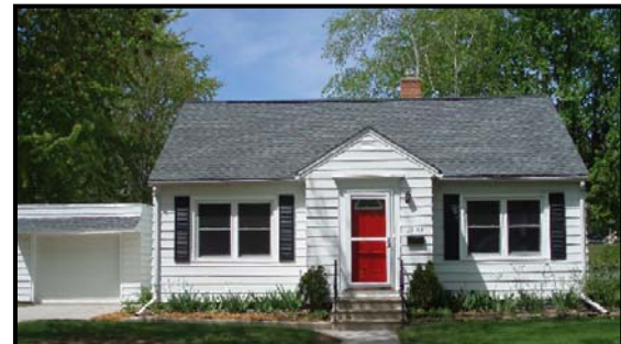
2044 12 th Street – After Rehabilitation
