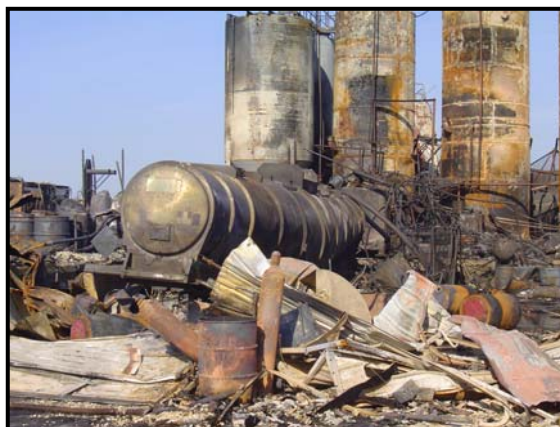
WRR Fire – Haz Mat team responded & mitigated
