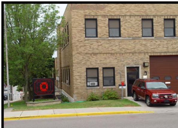
Fire Station #2 with Administrative Offices 216 South Dewey Street
