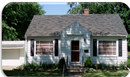
2044 12 th Street – Before Rehabilitation
