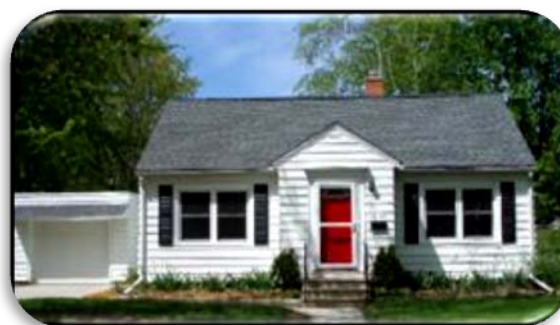
2044 12 th Street – After Rehabilitation
