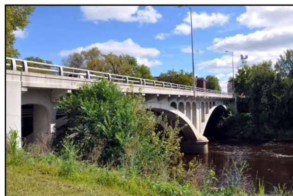
Dewey Street Bridge
