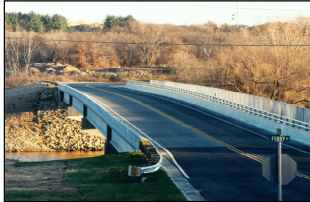
Short Street Bridge built in 2000
