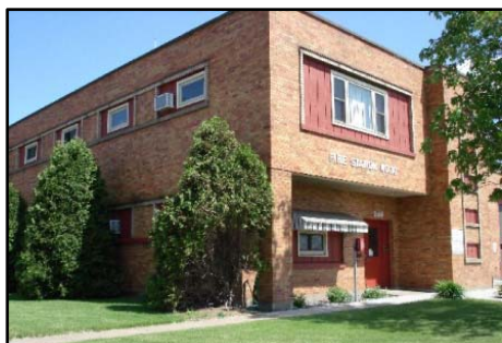
Fire Station No. 10, 559 North Hastings Way
