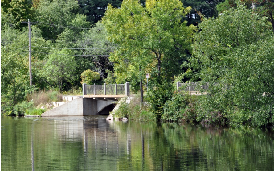
Lake Street Causeway Bridge
