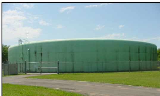
Mt. Washington ground storage reservoir prior to recoating in 2009
