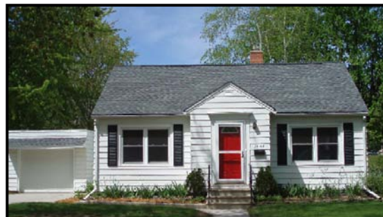
2044 12 th Street – After Rehabilitation
