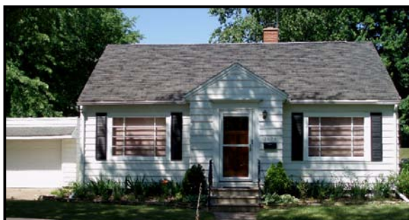
2044 12 th Street – Before Rehabilitation
