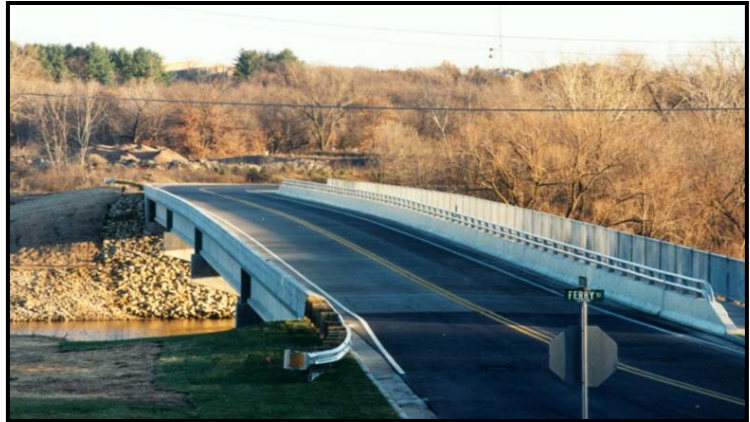
Short Street Bridge built in 2000
