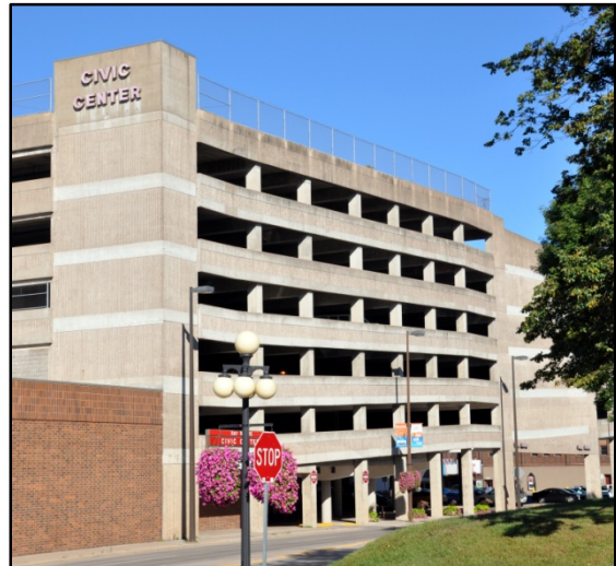
Civic Center Parking Ramp on Farwell Street
