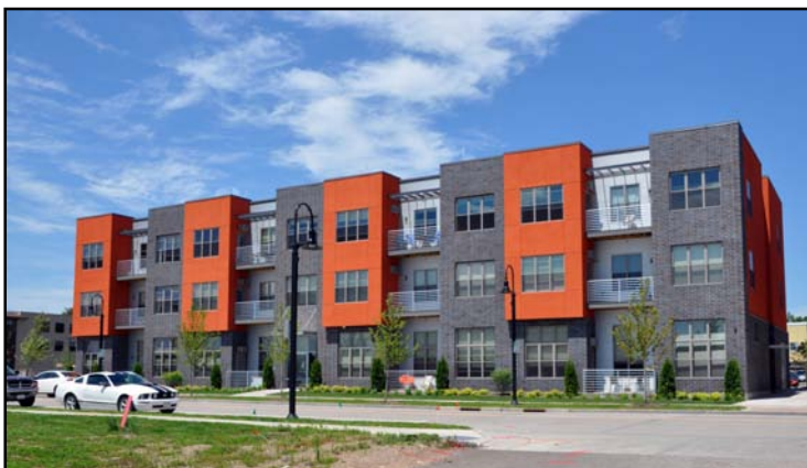
Phoenix Park Apartments, 312 Wisconsin Street, above and 315 Riverfront Terrace, right
