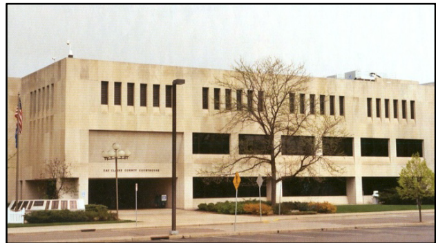
Eau Claire County Courthouse prior to construction of the new jail
