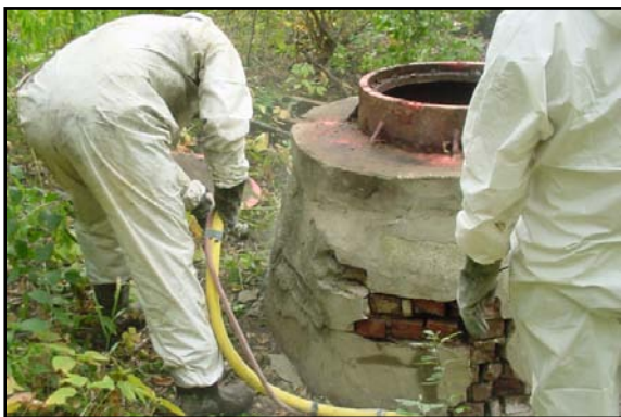
Chippewa River Sanitary Sewer Structure Reconditioning
