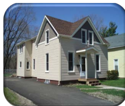
312 9th Street – After Rehabilitation
