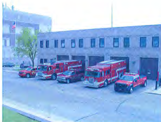
Fire Station #2 with Administrative Offices 216 South Dewey Street
