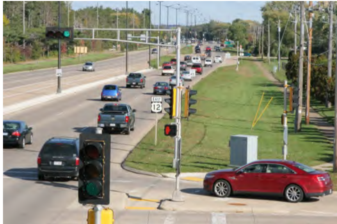
Access management standards promote traffic safety and flow by separating intersections or driveways along a road according to the type of road, its traffic volume, traffic speed and adjacent land uses.
