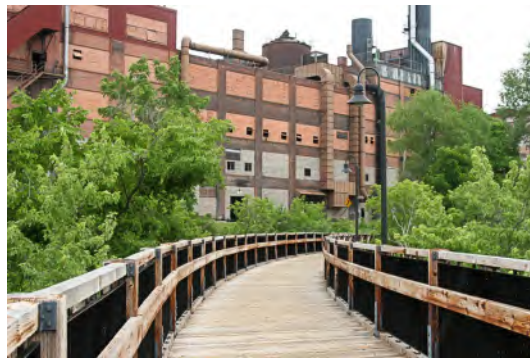
Banbury Place and the S Bridge
