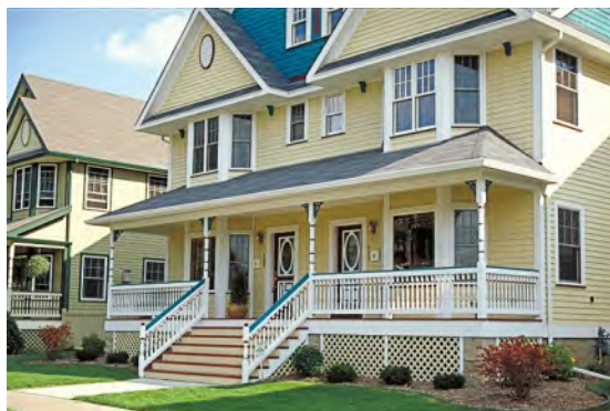
Infill and replacement housing, particularly attached units, should respect its neighbors, particularly in terms of garage placement.
