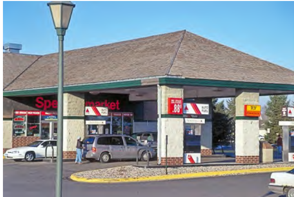
A convenience store with recessed canopy lights over the gasoline pump islands.
