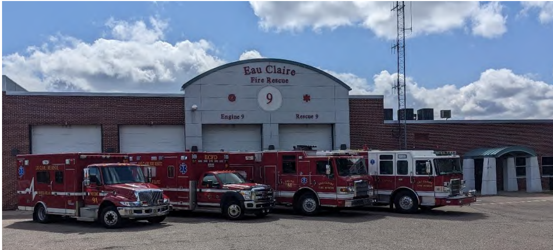
Fire Station 9—3611 Campus Road
