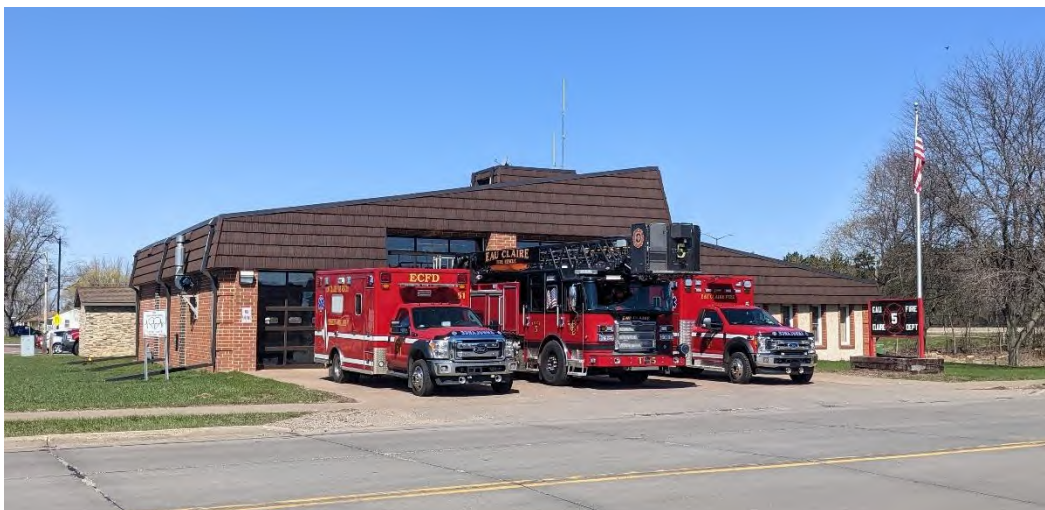
Fire Station 5—2500 Patton Street
