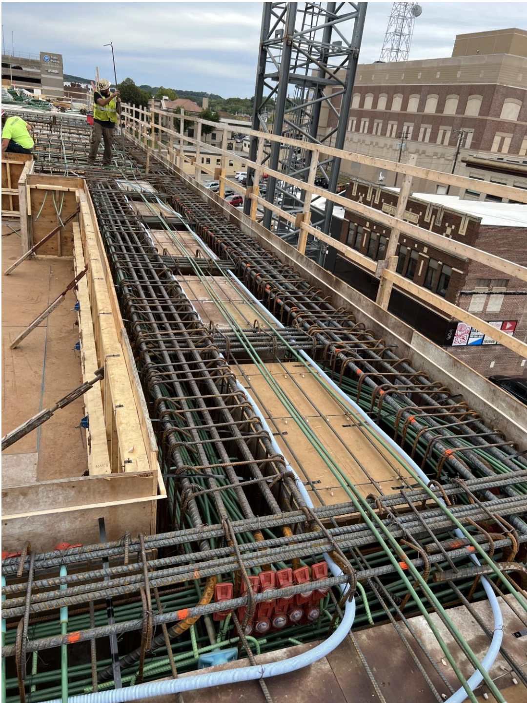
Photo 2 –PT Tendons and beams being laid out along Grid A
