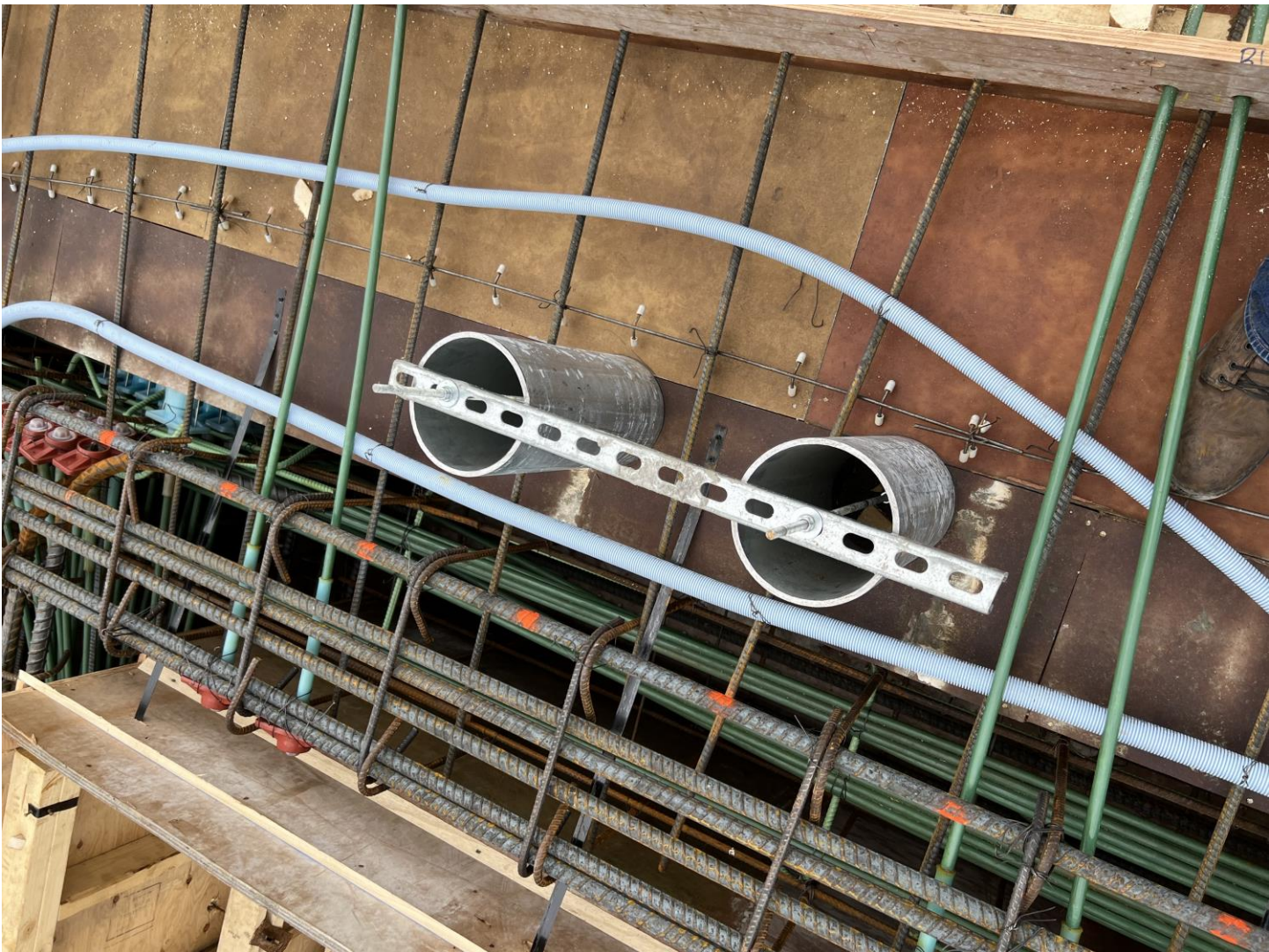
Photo 4 – Sleeves along Stair Core at Gridline A
