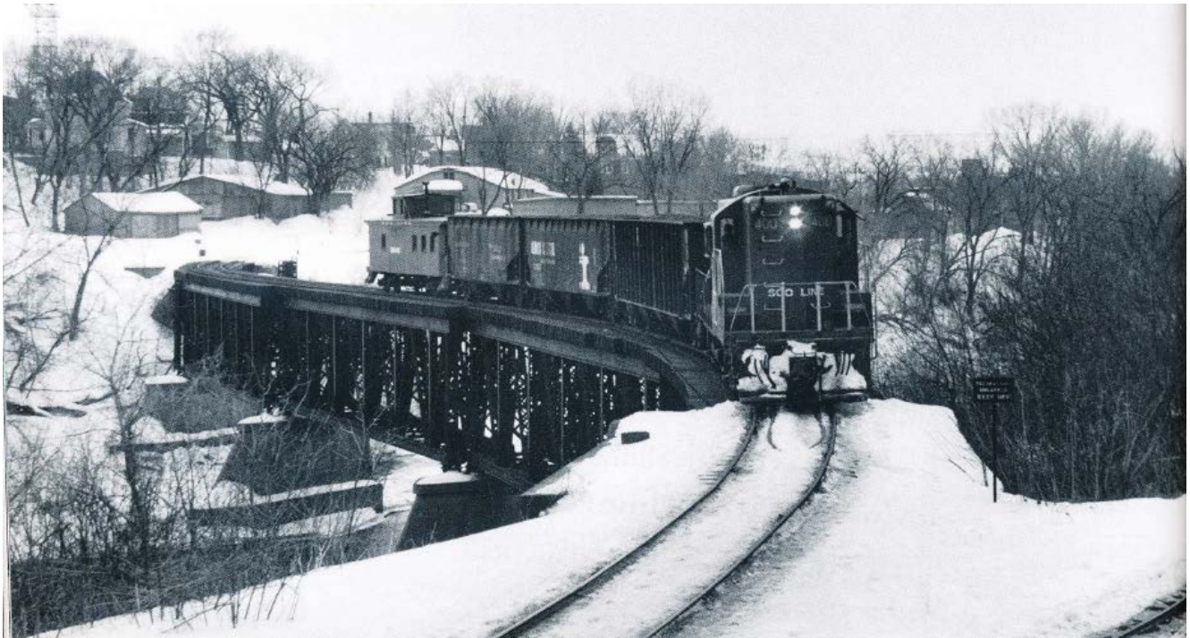
Figure 5: Figure 2: Soo Line Railroad Bridge, ca. unknown, Chippewa Valley Museum Collection, Eau Claire, Wisconsin.
