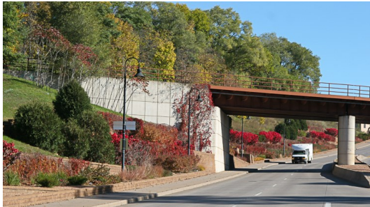
Birch Street at the Union Pacific Railroad bridge
