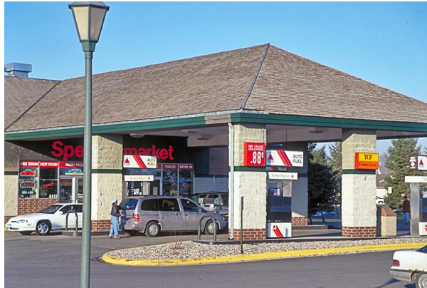
A convenience store with recessed canopy lights over the gasoline pump islands.
