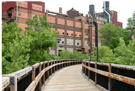
Banbury Place and the S Bridge
