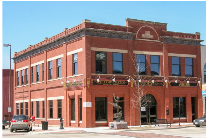
A fine example of commercial architecture, restoration and re-use in downtown.
