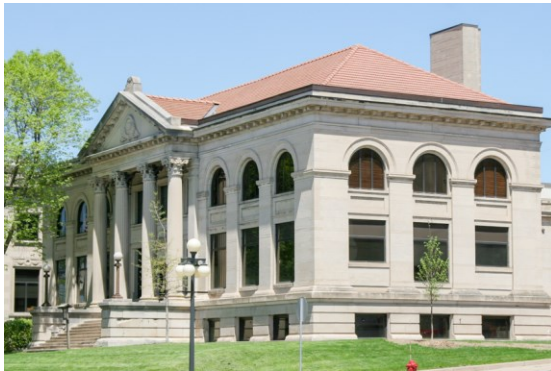
The Eau Claire City Hall is an adaptive re-use of an architecturally-significant library building.
