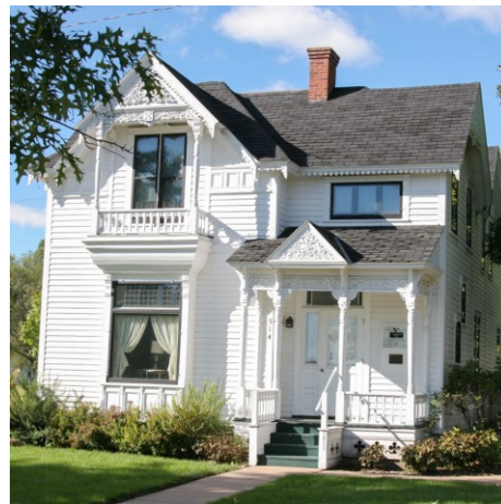
The Waldemar Ager house was saved and relocated for use as an historic museum and educational center.
