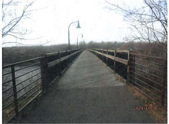
East Approach Looking West
