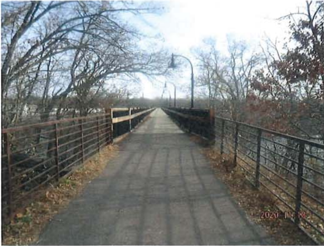
West Approach Looking East
