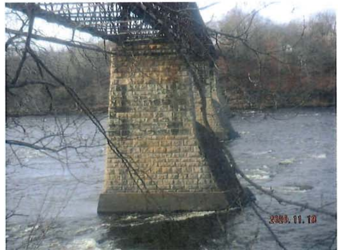
East Face of Pier 4
