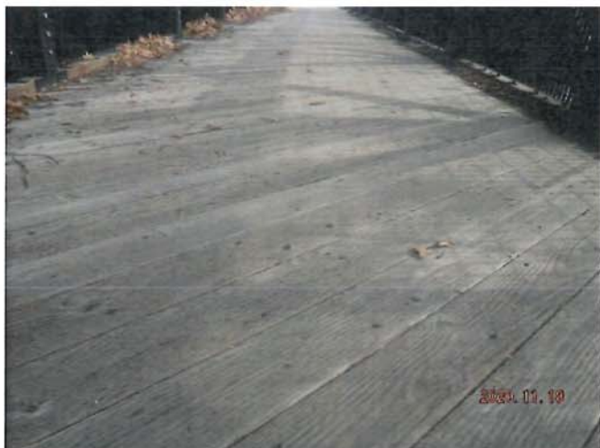
Typical Deck Condition
