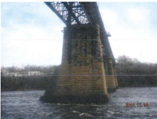
West Face of Pier 2
