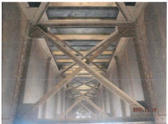
East Span Deck Underside
