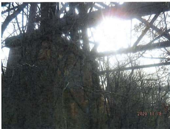
West Face of Pier 5
