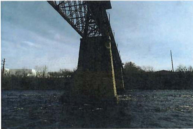
West Face of Pier 3
