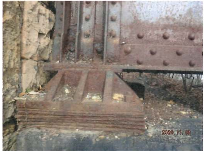
Typical Bearing at West Abutment
