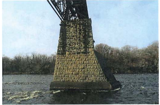
East Face of Pier 3
