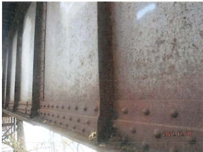
Typical Span 1 Girder Condition
