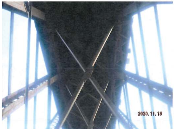
Typical Deck Underside Span 2, 3 and 4
