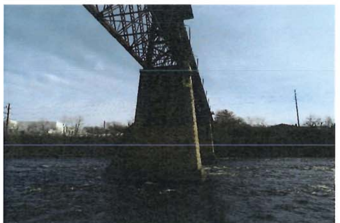
East Face of Pier 2
