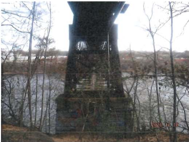
West Face of Pier 1
