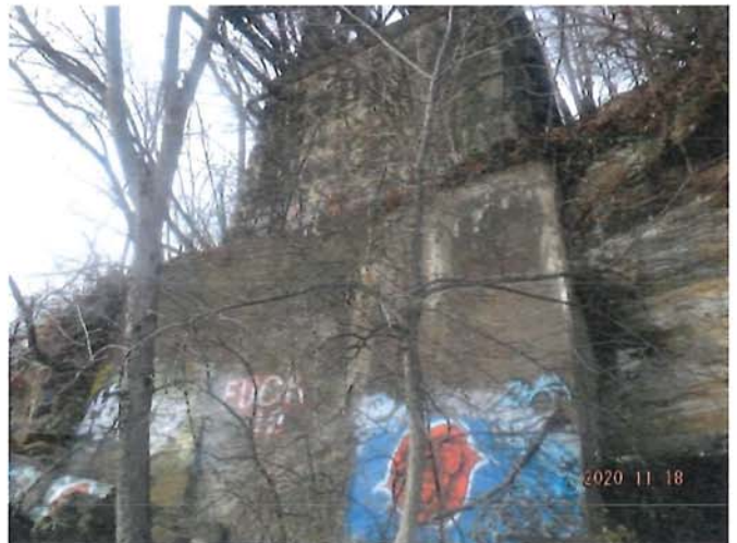
East Face of Pier 1
