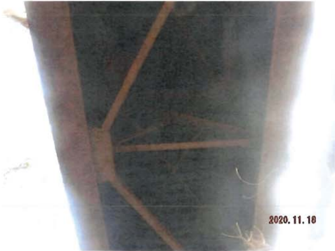
Typical Deck Underside Span 1
