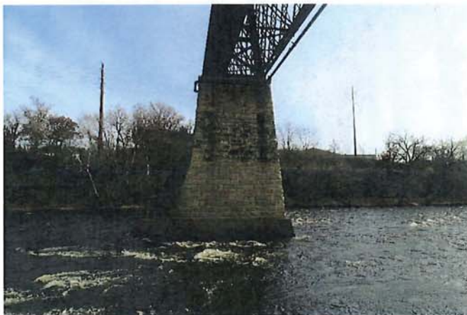
West Face of Pier 4
