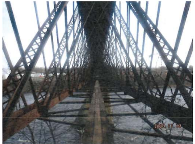
Looking East Through Span 2
