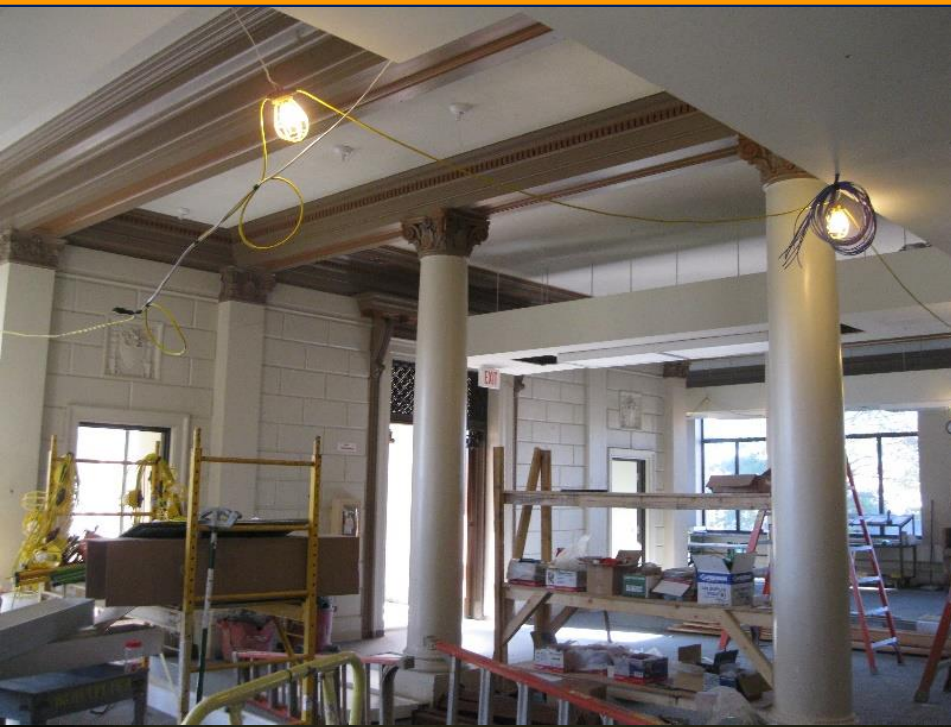
City Inspection and Planning Offices pre-construction
