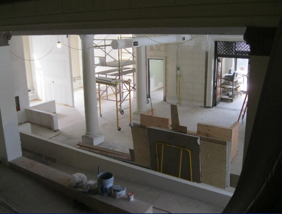
City Inspection and Planning Offices during construction
