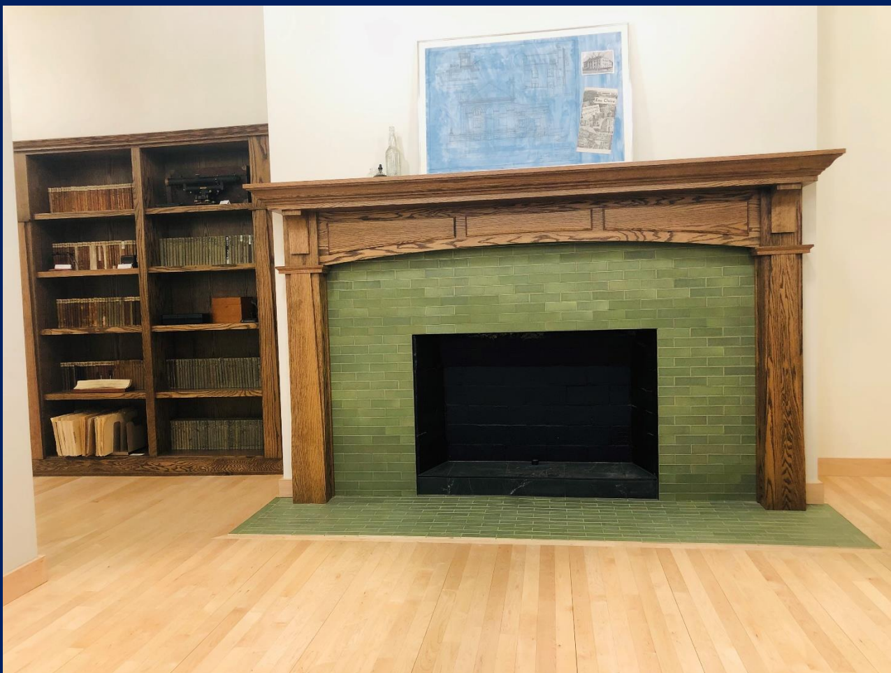
Restored second level fireplace with replica tile
