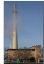
UW-Eau Claire's Coal-fired Power Plant
