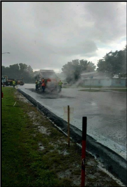
Asphalt Hotmix Patching
