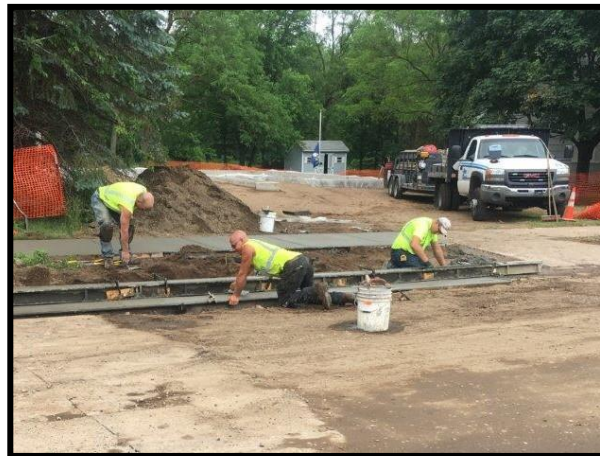
Concrete Curb and Gutter Replacement
