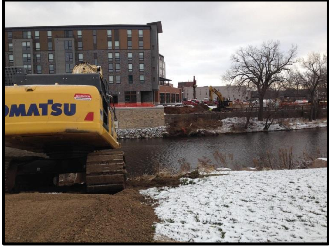
Utility Siphon Repair
