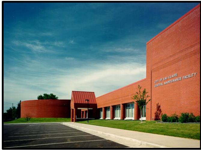
Central Maintenance Facility
