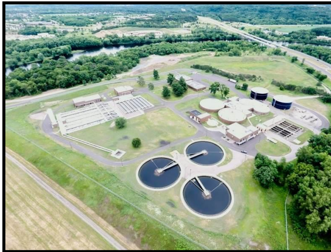
Wastewater Treatment Plant
