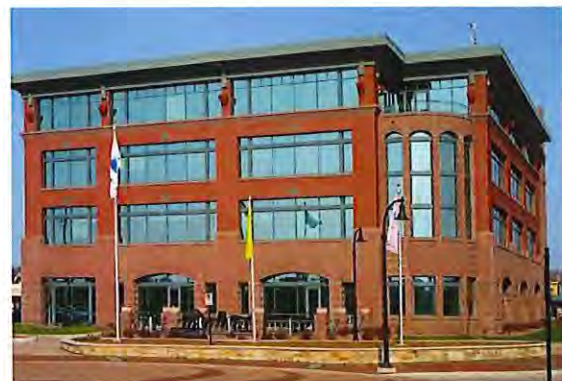
The RCU headquarters is an example of a building along the waterfront that respects and enhances its setting.
