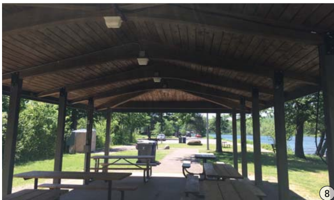
1.8 Views inside the shelter
