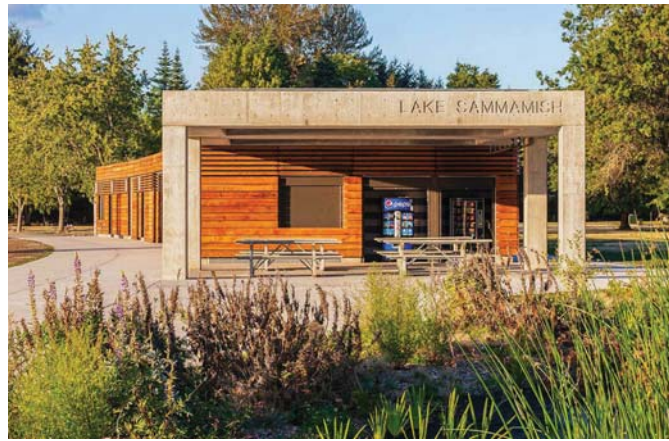
4.30 Renovated beach house with ground shelter
