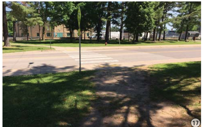
1.24 Carson Park Drive crossing from CVR to the baseball field
