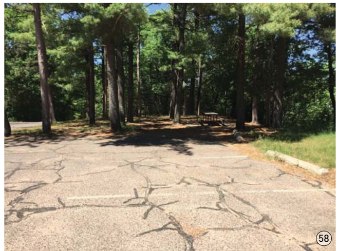
1.66 Picnic area and parking at point
