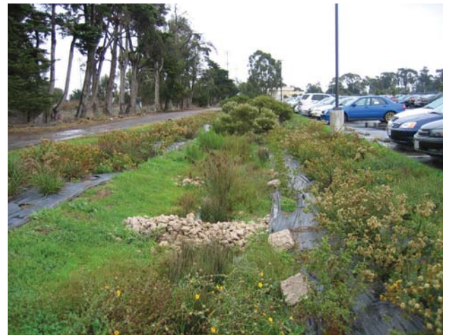
4.2 Bioswale on edge of a parking lot
