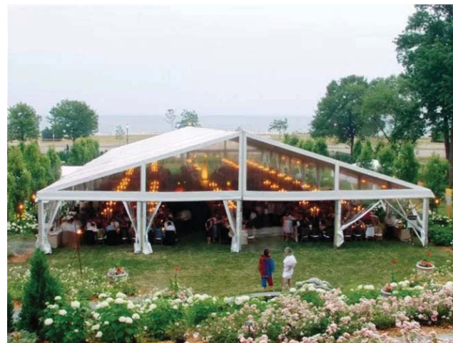
4.14 Portable clear span tent structure
