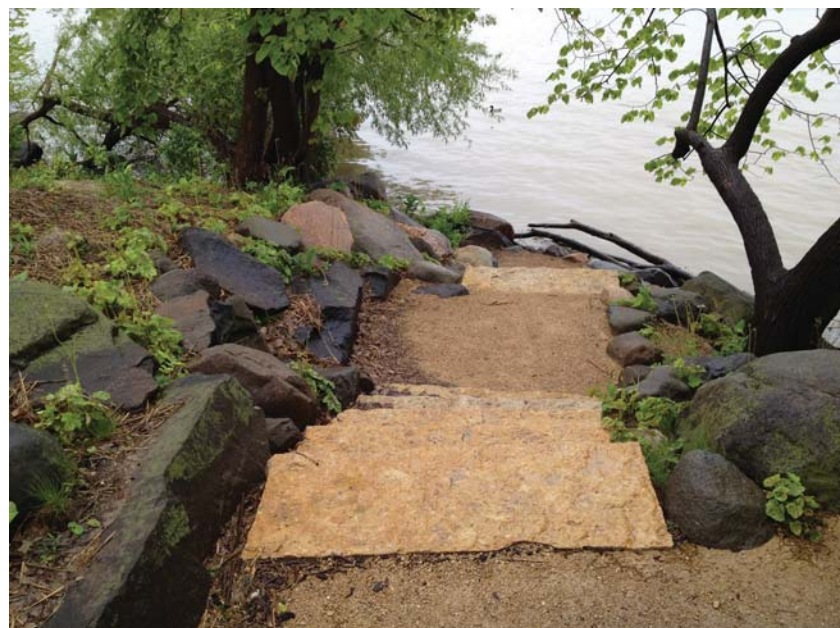
4.23 Natural stone rip-rap shoreline stabilization 4.24 Natural stone steps and crushed stone trail along a shoreline
