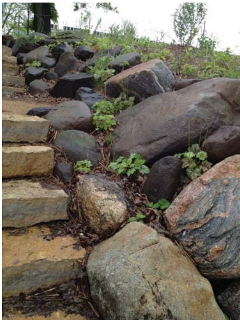
4.23 Natural stone rip-rap shoreline stabilization 4.24 Natural stone steps and crushed stone trail along a shoreline
