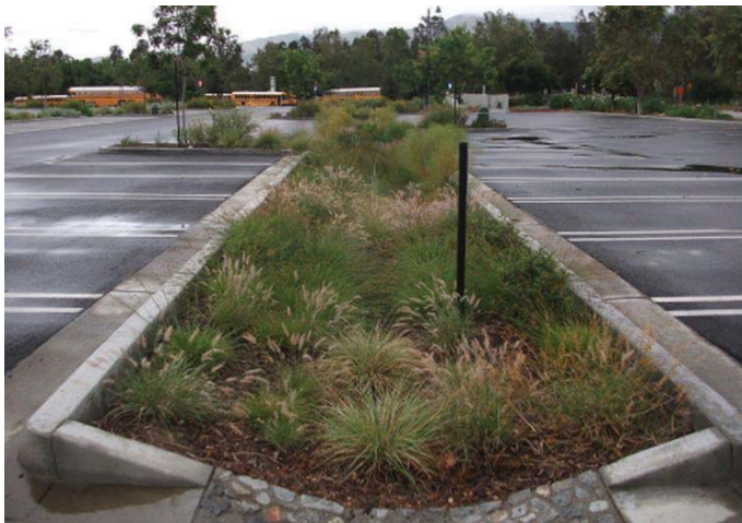
4.1 Bioswale in the interior of a parking lot
