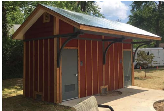
4.5 Vault restroom structure
