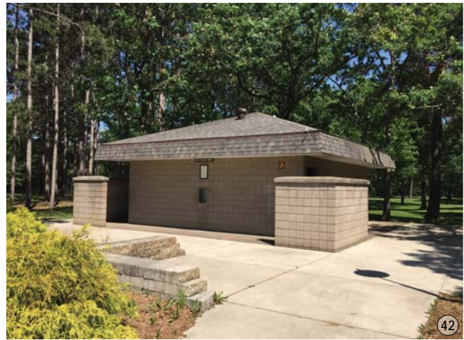
1.50 Restroom building near Pine Pavilion
