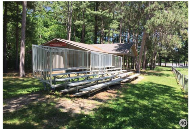
1.48 Bleachers at the horseshoe courts
