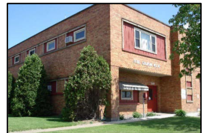
Fire Station No 10, 559 North Hastings Way
