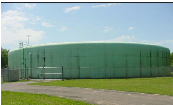
Mt. Washington ground storage reservoir prior to recoating (left) and after exterior recoating in 2009 (right). Interior painting of this reservoir is scheduled for 2013.
