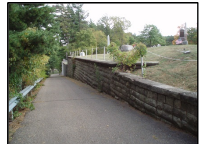
Forest Hill Retaining Wall
