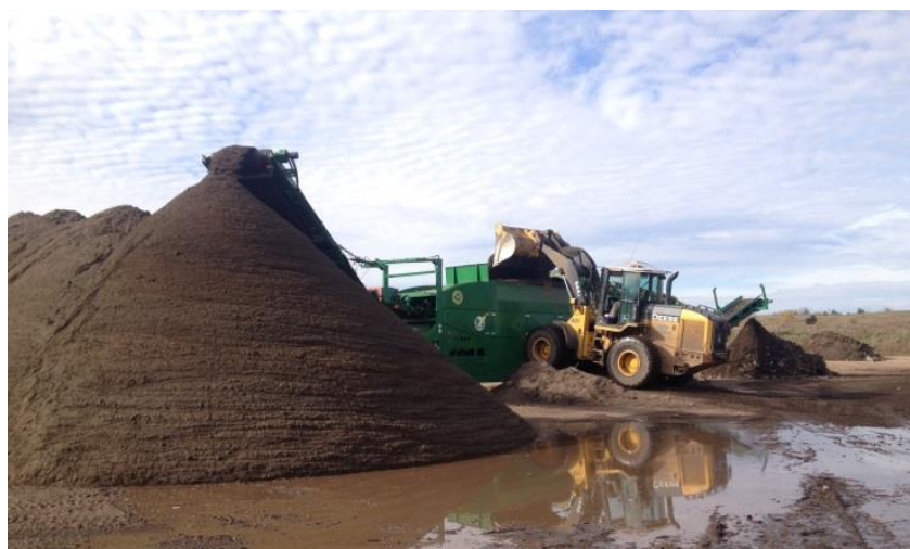
Screened street sweepings for reuse in Jeffers Road Brush Site berms
