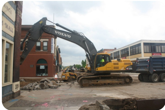
Street reconstruction on Barstow Street
