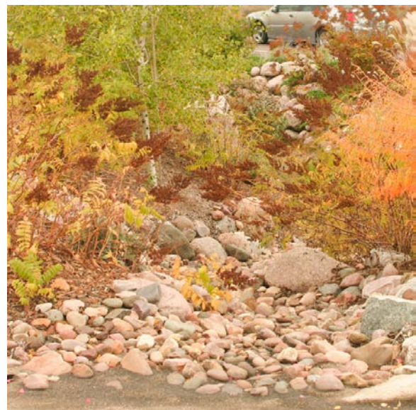
An example of a vegetated island in a parking lot that catches and treats runoff polluted with salt, sand and automotive fluids.
