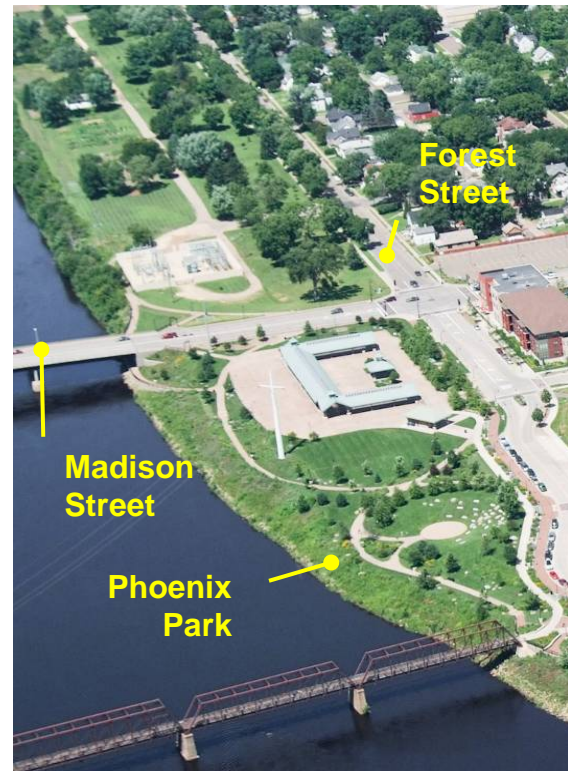
The floodplain west of Forest Street and Riverview Terrace has been cleared and transformed into park.
