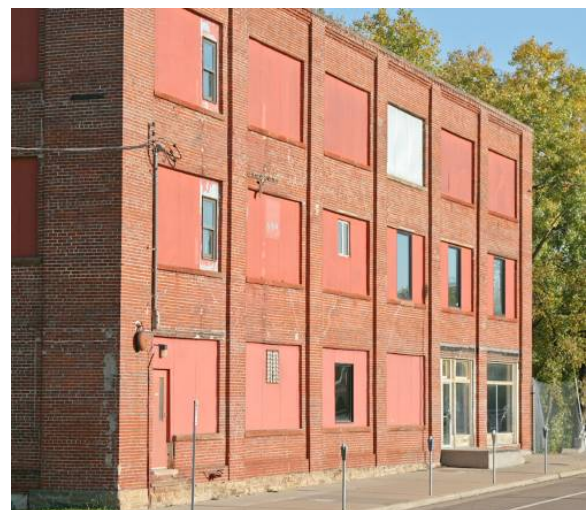
Adaptive re-use of waterfront industrial buildings helps interpret local history and provides a sense of the early role of the rivers.
