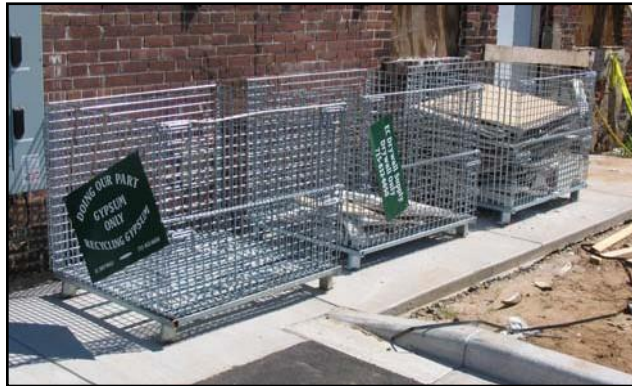
Recovered Gypsum Board at an Eau Claire construction site
