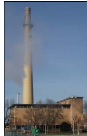
UW-Eau Claire's Coal-fired Power Plant
